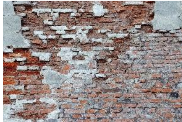
Lapisan finishing lepas
