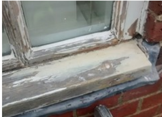
Lapisan finishing lepas
