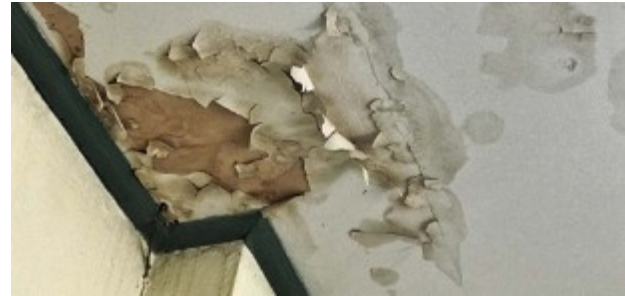
Lapisan finishing lepas
